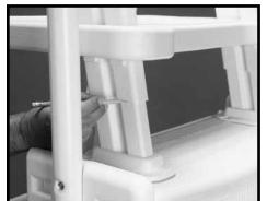
**#2:** Position the ladder so the Mounting Blocks sit flat. Using a pencil, mark the height on the Mounting Block Tubes. *NOTE: If necessary you may need to cut down the Mounting Block Rails with a hacksaw.*
