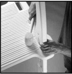
**#3:** Stand up the assembly and using a rubber mallet tap the Platform down until seated on the lugs on the Side Rails. IT MAY REQUIRE SEVERAL HARD BLOWS WITH A RUBBER MALLET TO SEAT THE PLATFORM ALL THE WAY DOWN ONTO LUGS.
