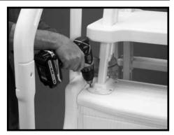
**#4:** Position the ladder over the pool step with the Mounting Blocks sitting flat on the top tread. Center the ladder side-to-side and align the back of the Mounting Blocks next to the groove in the back of the Platform as shown. Attach using four #10 x 3/4" self-tapping screws in each Mounting Block.
